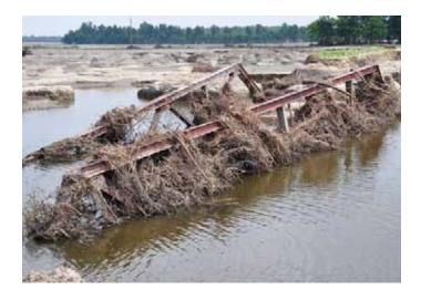
I suppose I shouldn't say the bridge is "missing." It's still located in the same spot, but has been turned into a mangled mass of metal, half-buried in debris and water. What was once a small drainage ditch has been widened into a river. When the surge came, the bridge didn't stand a chance.
